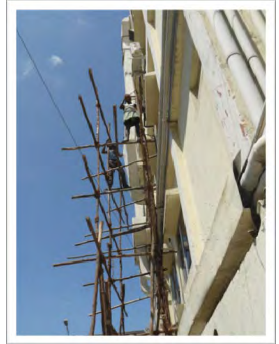
FIGURE 6: EXTERIOR RENOVATION OF A HOSPITAL TREATING INTERNATIONAL PATIENTS, INDIA. 2010.
