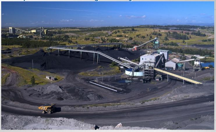
Coal-handling and preparation plant with maximum feed capacity of 4.5 Mtpa of ROM coal, producing semi-soft metallurgical coal and thermal product coal, which will be placed in separate product coal stockpiles
